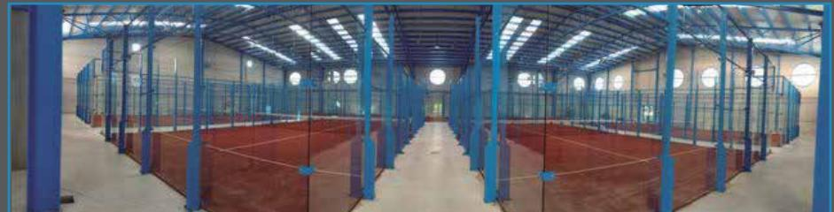
The main structure of the court is made of 100x60x3mm and 80x60x2 laminated / hot rolled steel profiles with quality S-275-JR and S-235-JR.
