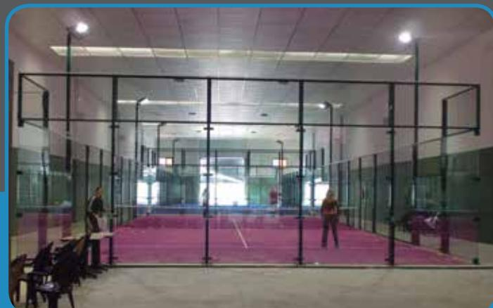
The main structure of the court is made of 100x60x2mm and 60x60x2 laminated / hot rolled steel profiles with quality S-275-JR and S-235-JR.
