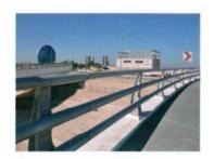
The **VGAN 300** aluminium parapet is a modular design, consisting of 3 horizontal rail sections located to supporting posts. The system is 1070mm high and is made from special grade aluminium to meet the demands of the larger vehicle.
