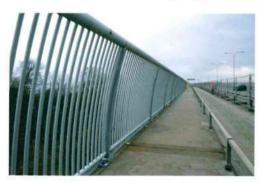
A special tubular design for the Erskine bridge in Scotland (pictured left) provides a high level of protection. The system was provided with enhanced galvanising to increase its corrosion protection. Each standard panel was 2.4m high by 4m long.
